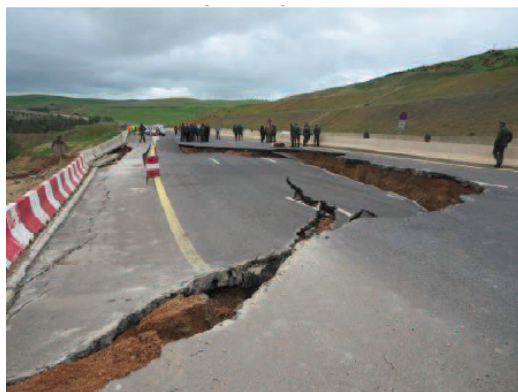
Fig. 1. Deformation of the pavement of highway at Pk52.
