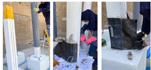
Fig. 7. Circularization and CFRP-EB technique.
