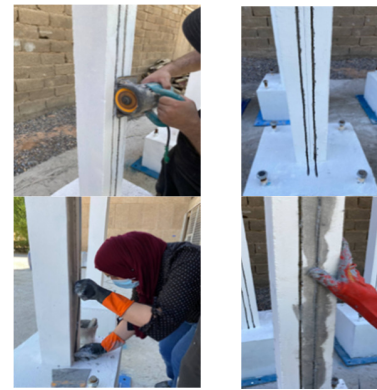
Fig. 6. NSM-CFRP technique procedure.
