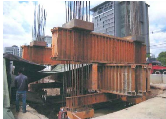
Fig. 8. Static pile load test.
