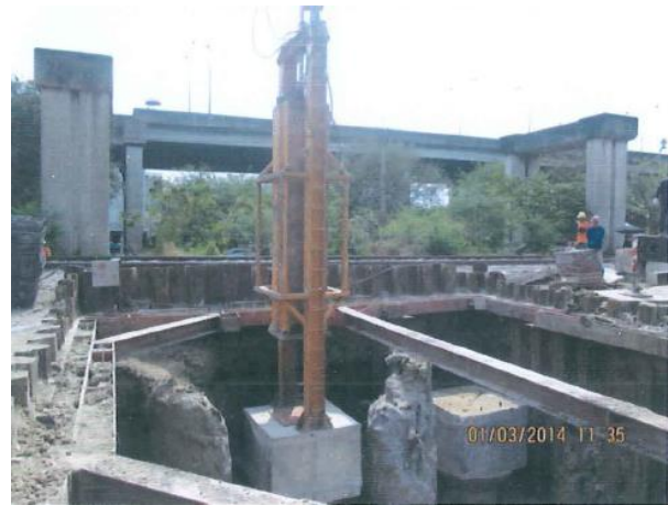
Fig. 6. Dynamic pile load test.
