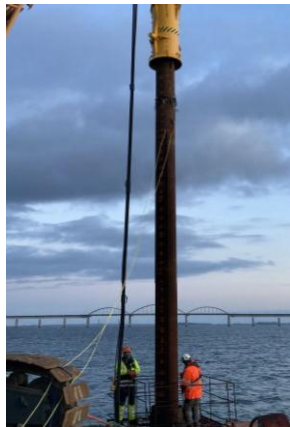
Fig. 1. Follower used for piling activities with above-water instrumentation
