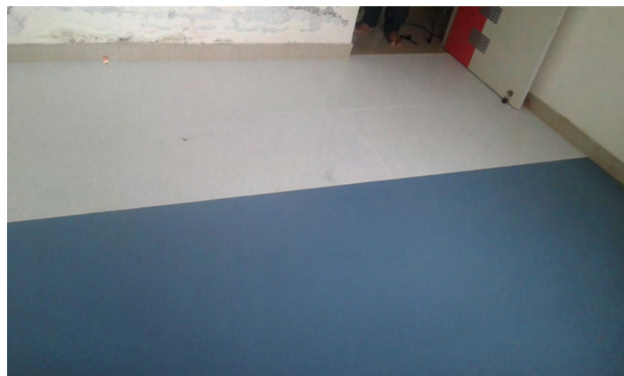
Figure 8. Final installed conductive tile and antistatic mat flooring
