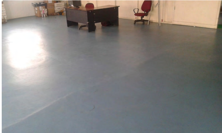
Figure 3. Antistatic Mat Provision At D.C.P.L with grounding
