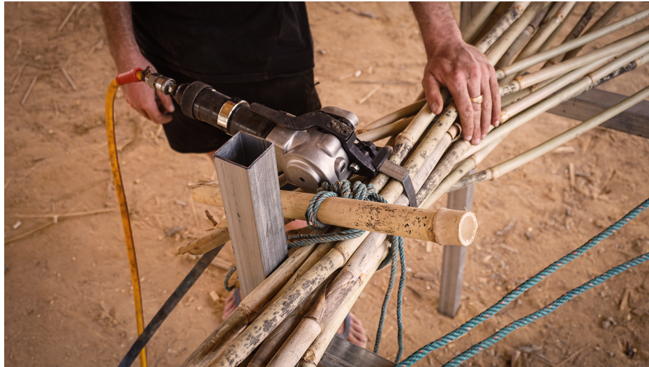
Figure 7: Pneumatic strapping with galvanized steel straps
