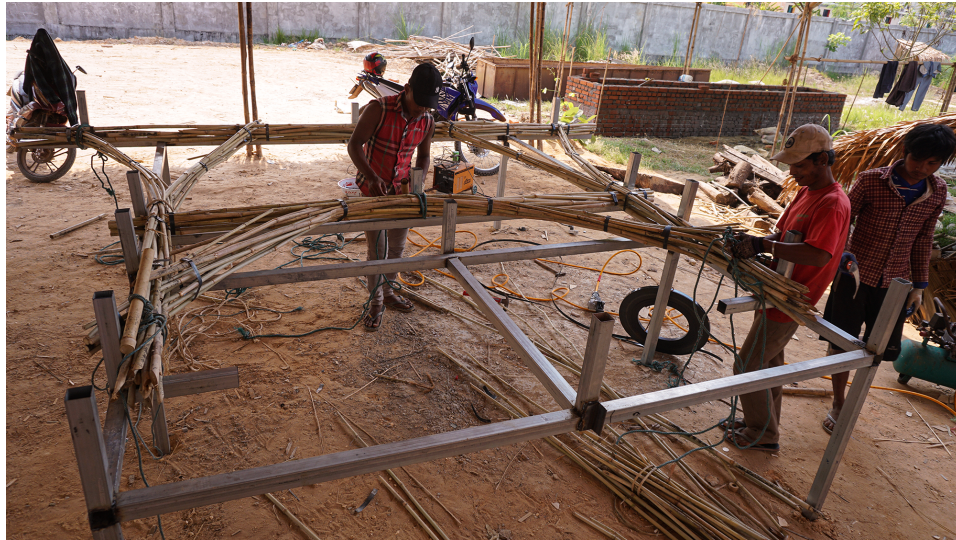
Figure 6: Fabrication of the frame on the metal framework
