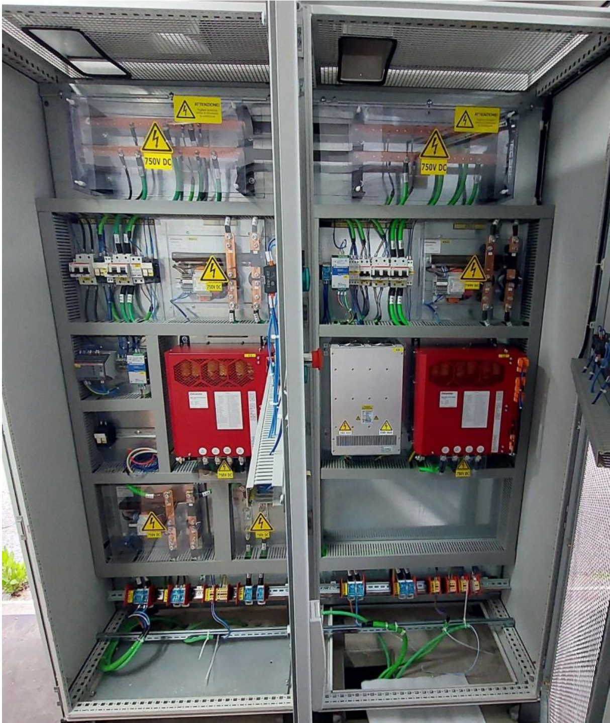
Figure 41: Italian pilot - storage and photovoltaic DC power supply.
