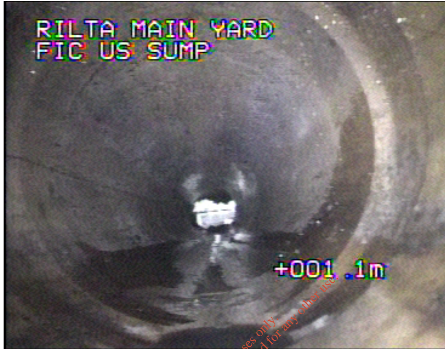
Photo: 19_3A, MPEG #: 280217_1, 00:00:27 1.1m, Open joint, medium
