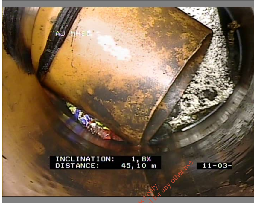
Photo: 8_14A, MPEG #: 280217_1, 00:13:29 45.49m, Connection other than junction, at 10 o'clock, diameter 100mm
