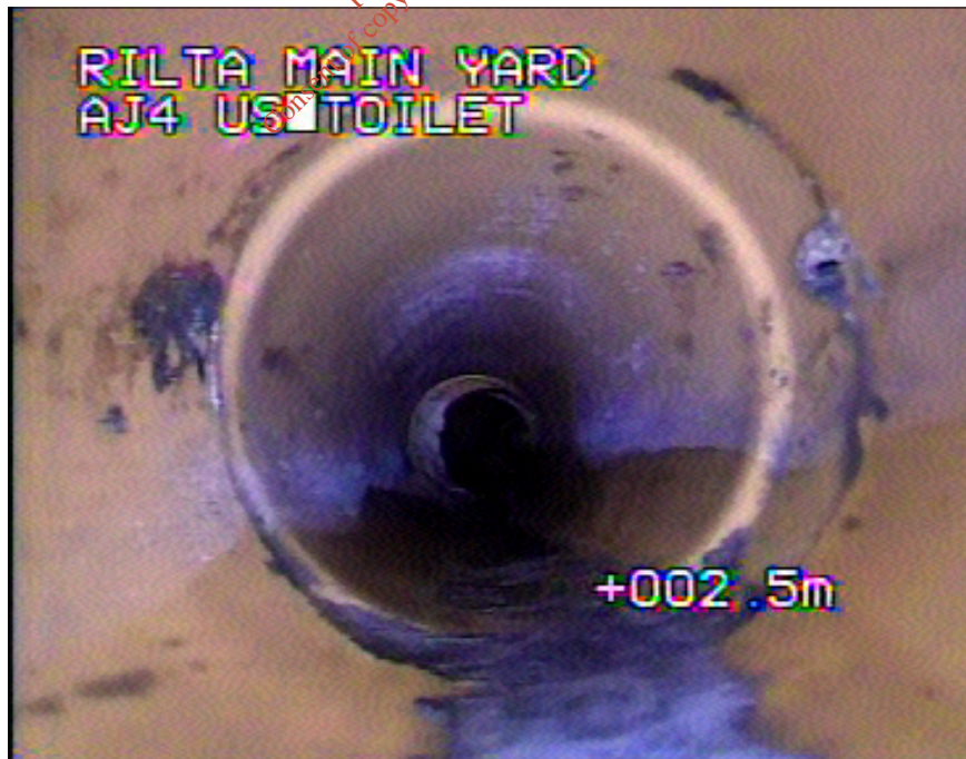
Photo: 13_4A, MPEG #: 280217_1, 00:00:36 2.5m, Open joint, medium
