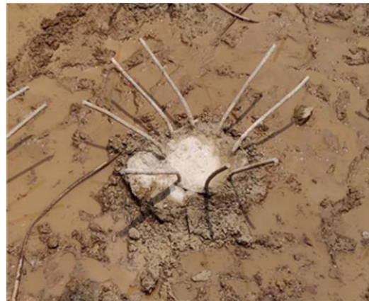
Fig. 2 Condition of prepared pile head
