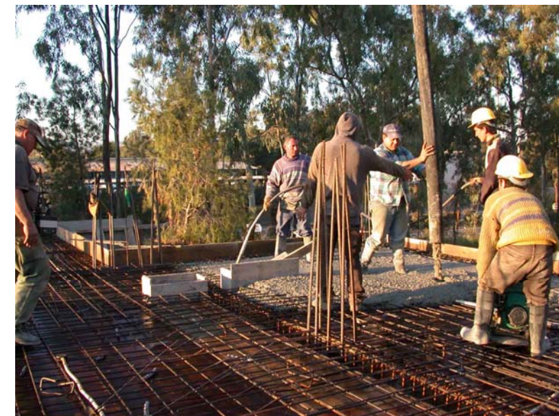
Figure 6.5: Concrete floor slab construction
