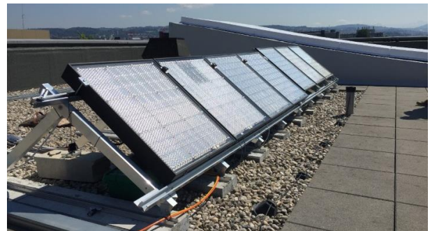
Fig. 1 A 1kW demo array of Insolight's micro-CPV product installed at EPFL in Lausanne, Switzerland. A subset of these modules has been in operation for over 1 year. Observe that these high-efficiency panels are installed south-facing and fixed-tilt using conventional flat-plate mounting hardware.
