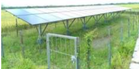
Figure 1. PV 11 kWp as a supply pump
