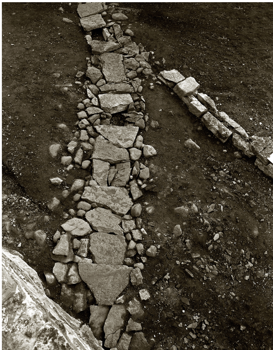
Figure 3. Secondary built closed drains could have been a good way to a drier indoor climate. Here is an example from the northeastern corner tower of the bishop's residence in Hamar. Source: Anno Domkirkeodden.
