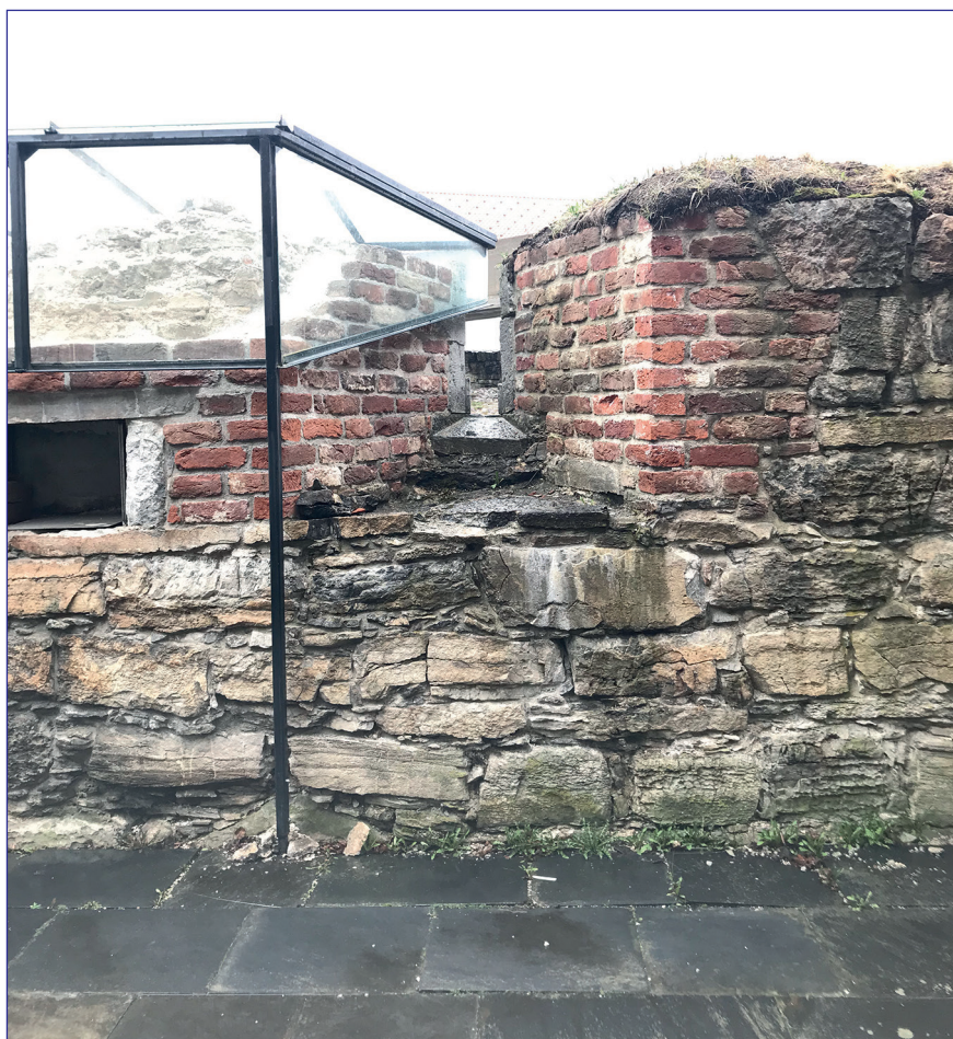
Figure 4. In eastern Norway brick use in rebuilding contributed to warmer dwellings. At the southern wing hall at Hamar, all openings were narrowed down in order to make warmth stay inside rooms. Source: Kristian Reinford.
