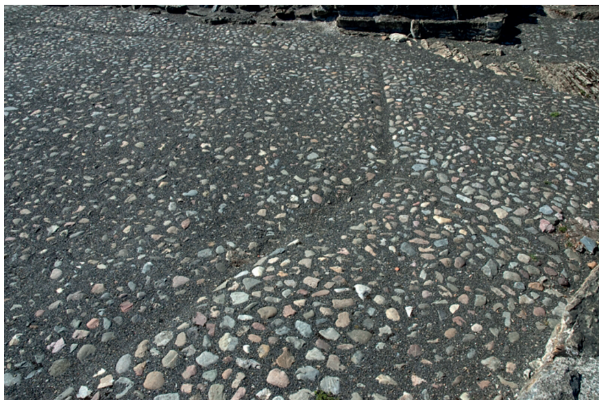
Figure 2. Inserting drains down into cobblestone floors to secure a drier courtyard was an architectural adaptation of the sixteenth century. Here as part of the Hamar bishop's residence. Source: Anno Domkirkeodden.
