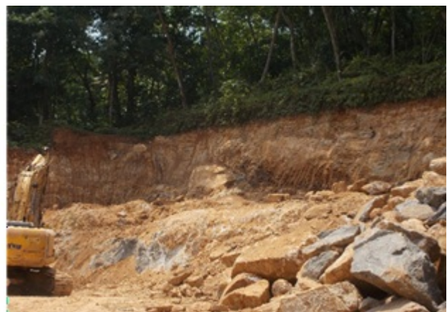
Fig. 7. (a) Contour terracing without a proper drainage system, and (b) development activities that could destabilise the slopes.
