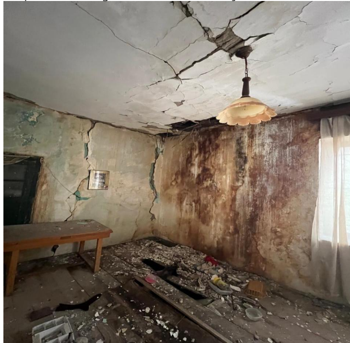
Figure 2. Building S2 severe damage on perimeter walls
