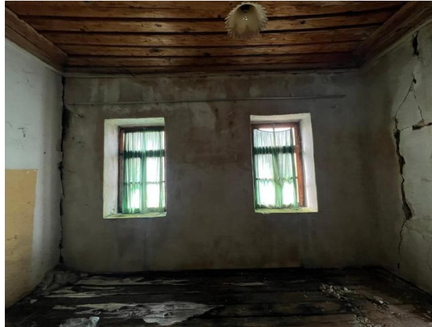
Figure 4. Building S2 lack of box behaviour
