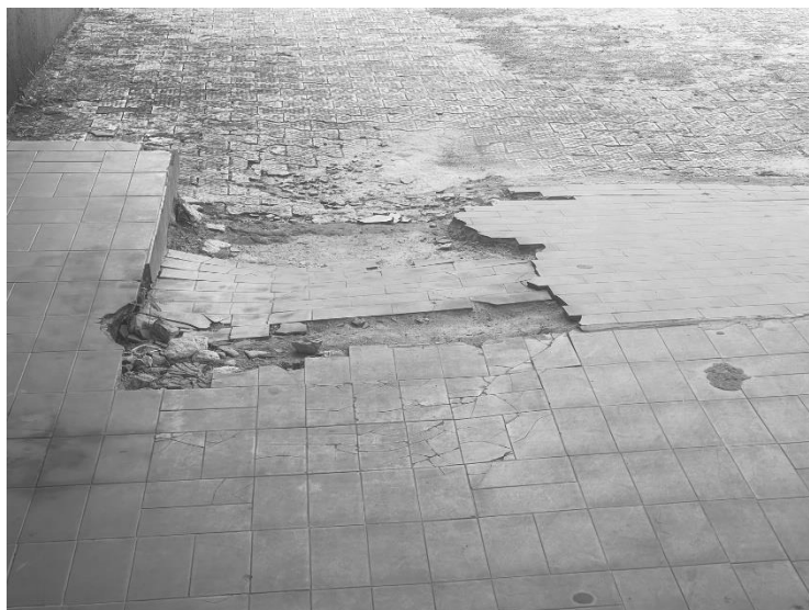
Figure 2: Detached and cracked floor tiles at the UNIBEN Bursary Office Building (Photographed and modified by K.J. Eweka 2025)
