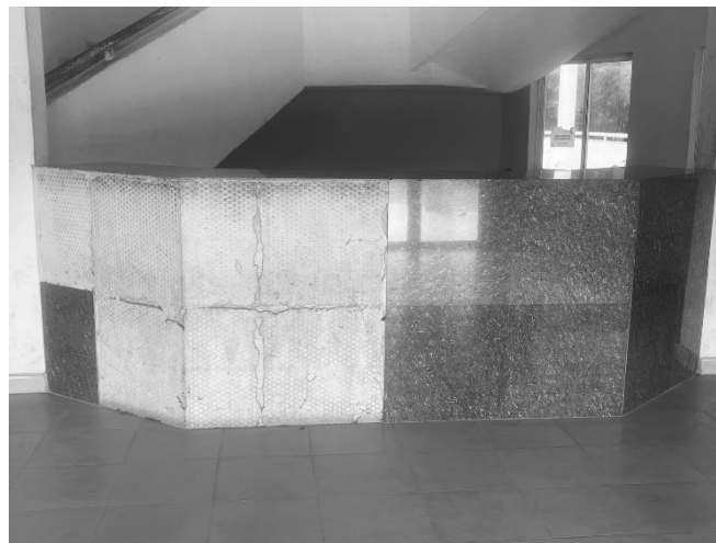
Figure 3: Poorly matched wall and floor tiles in the faculty's lobby (Photographed and modified by K.J. Eweka 2025)
