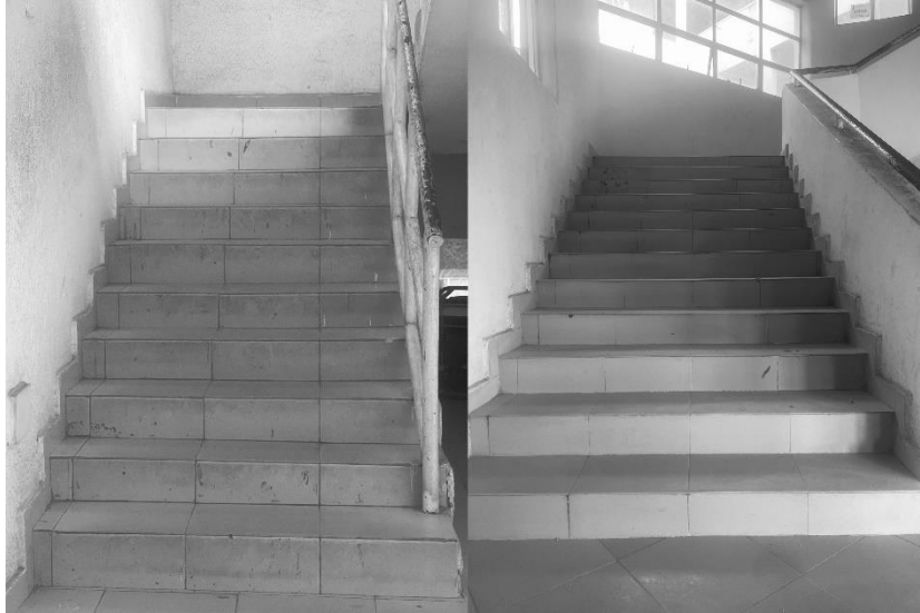
Figure 1: Slippery glossy tiles installed on staircases, Faculty of Environmental Sciences and the Bursary Office Building (Photo-montage and modified by K.J. Eweka 2025)
