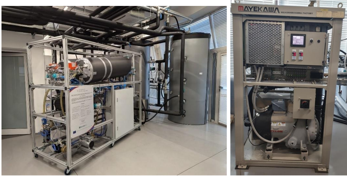
Figure 7 Sorption storage connected with Mayekawa CO2 Heat Pump in KEZO Research Centre
