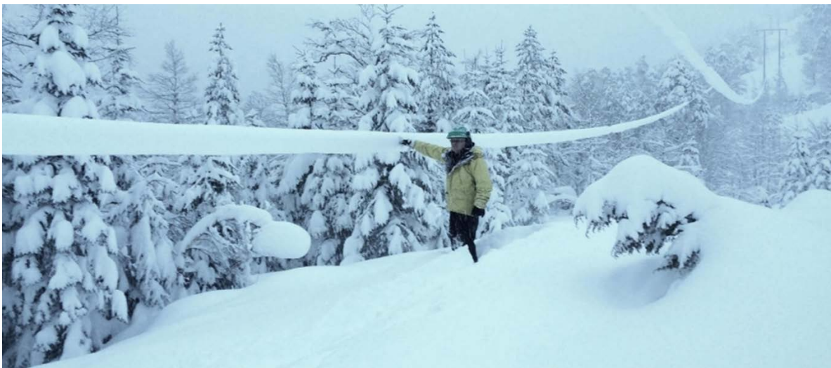
Figure 2: Wet snow accumulation on power lines (BKK Nett, Norway).
