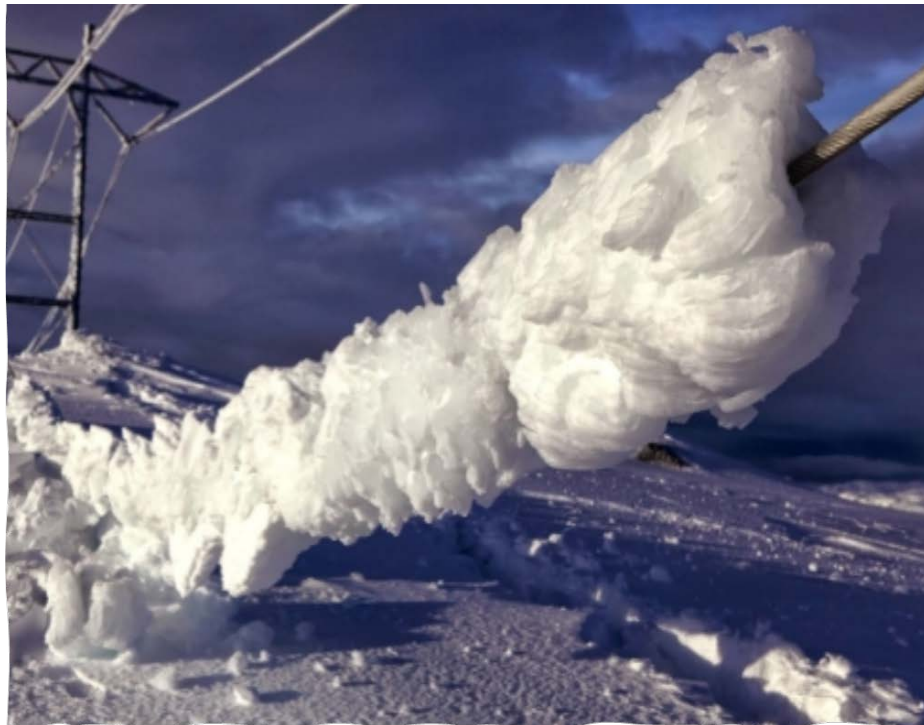
Figure 1: Atmospheric icing on electrical infrastructure in Ålvikfjellet, Norway (2013).
