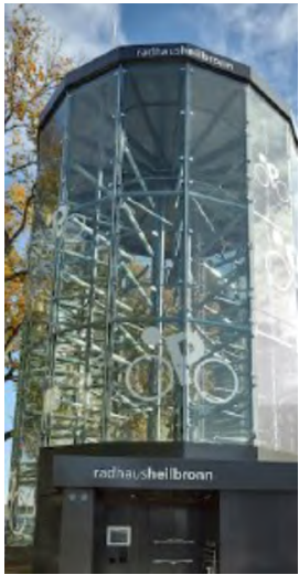
BIKE PARKING / Visible Bike Parking WÖHR system with glass skin
