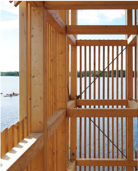
BUILD IN WOOD / Timber structure and timber facade of FSC-certified wood
