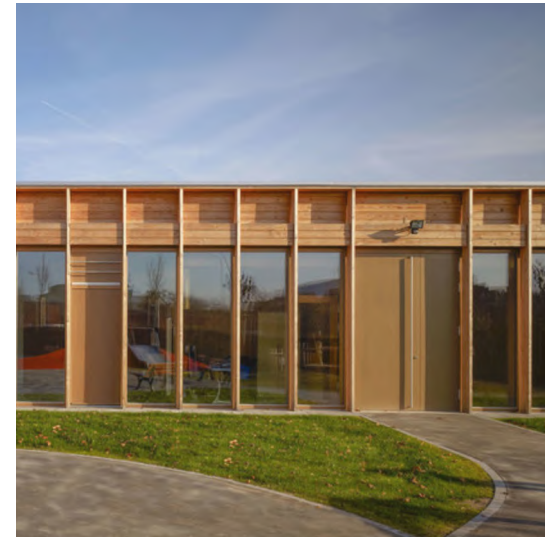
Modular façade solid/ openable modules
