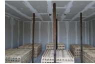
Non-combustible on all sides 2 x 25 mm gypsum cladding
