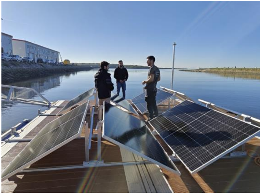
Figure 5.2 - Floating solar panels installed on the floating dock on the Ave River estuary.
