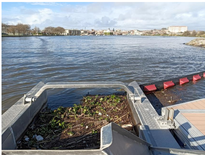
Figure 4.6 - Catchment System view from floating platform. Bubble curtain can be seen along the river in the top left corner of the picture. Source: TGBB.
