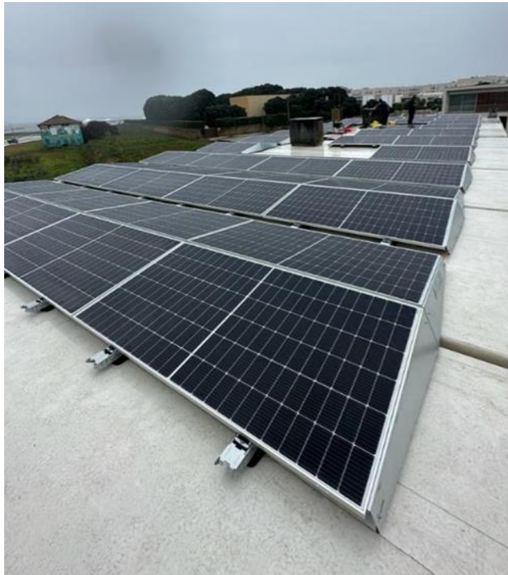
Figure 5.1 - Solar panels installed on the rooftop of the CMIA building.
