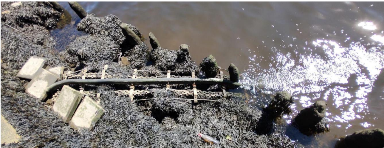
Figure 4.9 - At the northwest extremity of the Bubble Barrier, the bubble hoses would occasionally be exposed during low tide. The situation has been mitigated by shortening and repositioning.
