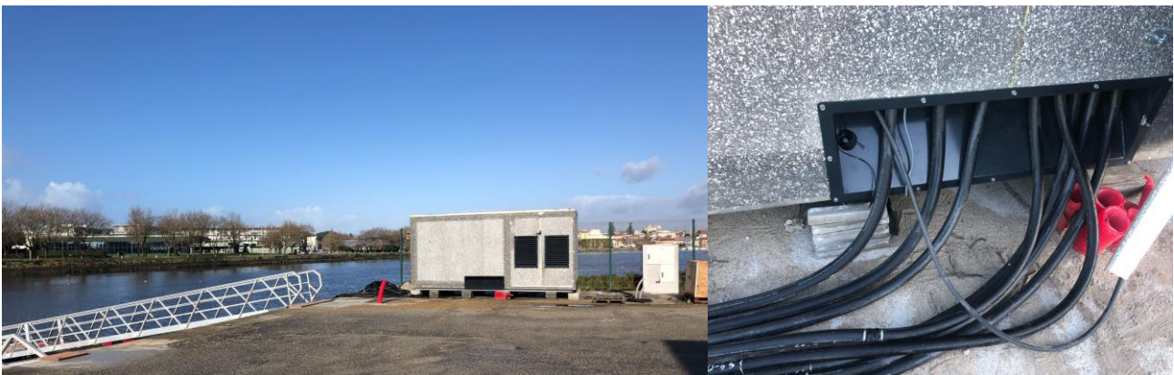
Figure 4.5 - Images from 15/12/2023, when the containerized compressor was placed at the right location and integrated into the Bubble Barrier. Source: TGBB.
