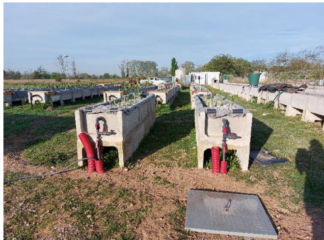
Figure 7. CW system (Montornès del Vallès WWTP)
