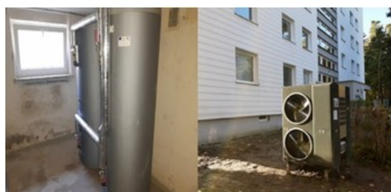
Figure 7. DHW (Domestic Hot Water) tanks and GSJ 46EVI HP in the Polish demonstration site
