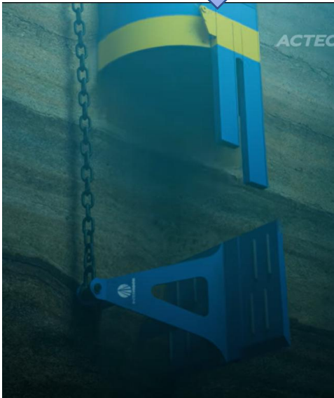
Suction embeded plate anchor (SEPLA) installation process
