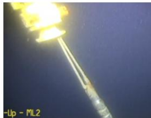
5. Pull using onboard winch
