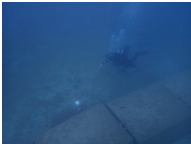
Fig. 4. Part of the 300m long wall protecting the canalisation overflow pipe in Valsaline bay with diver approaching a sensor location
