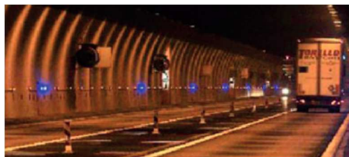
Fig. 3 blue marker lights in a tunnel (photo CETU)
