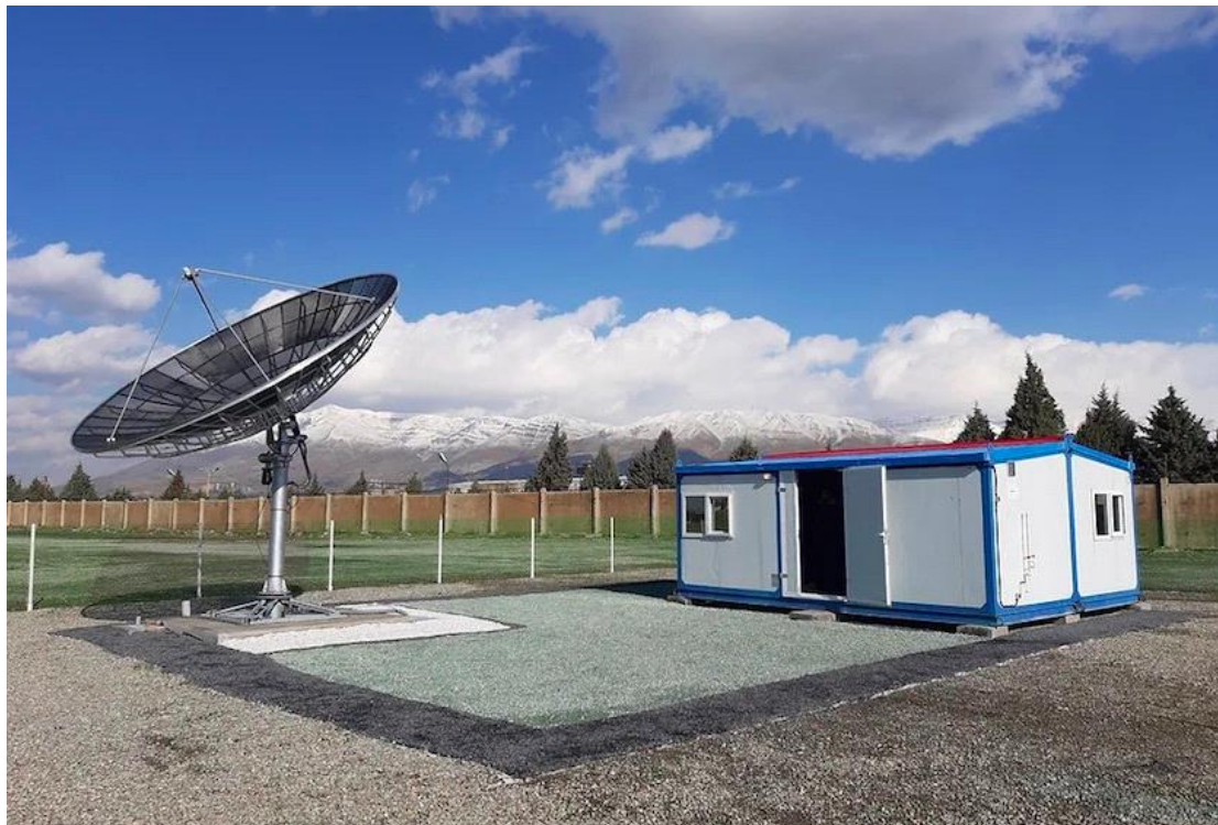
Figure 4-2: Poam Electronics 6m Mesh Reflector - motorized mount.
