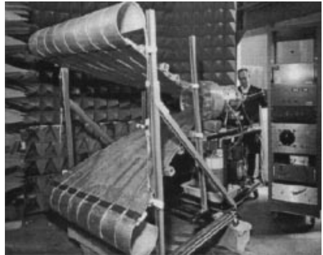
Fig. 2. H-2 with large TEM horn.
