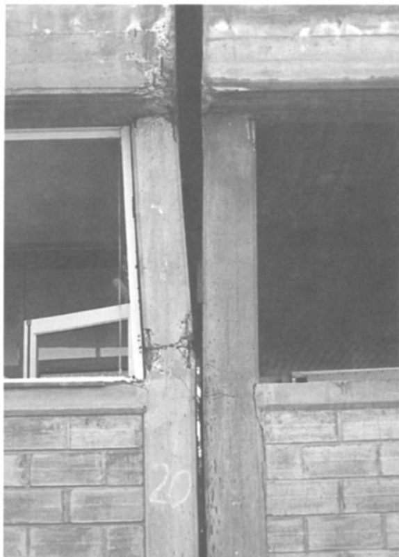
Fig. 13. Fractured and tilted column at the end of the damaged section of Escuela Normal building.
