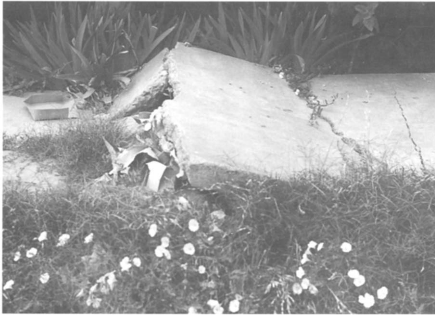
Fig. 14. Concrete side-walk buckled and shortened by about 130 mm due to compressional ground displacement on the Escuela Normal campus. (Location noted on Fig. 11.)
