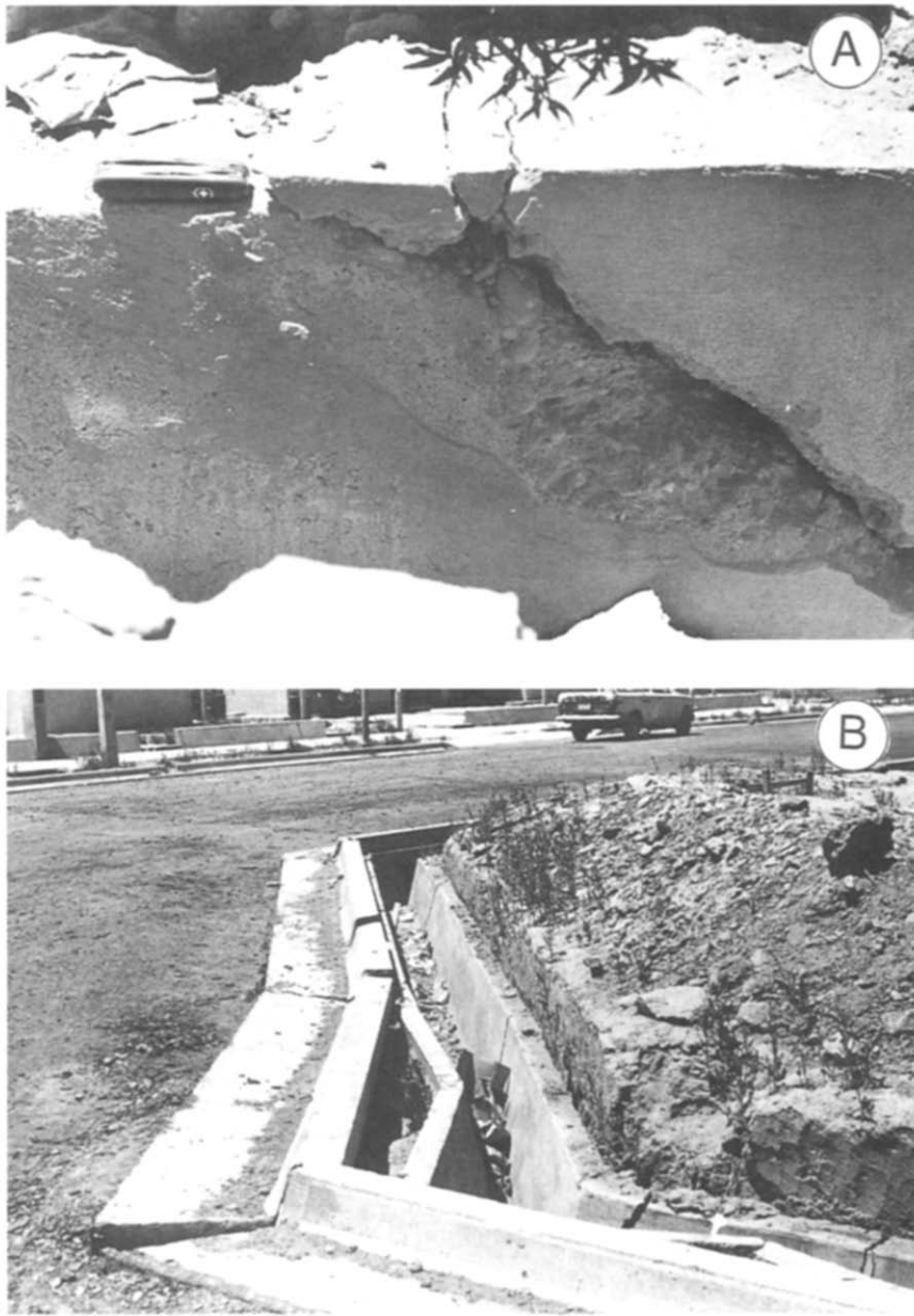
Fig. 6(A). Curb that was sheared and (B) canal linings that buckled due to compressional forces generated by liquefaction-induced ground oscillation and consequent impacts between mobile and immobile soil segments.
