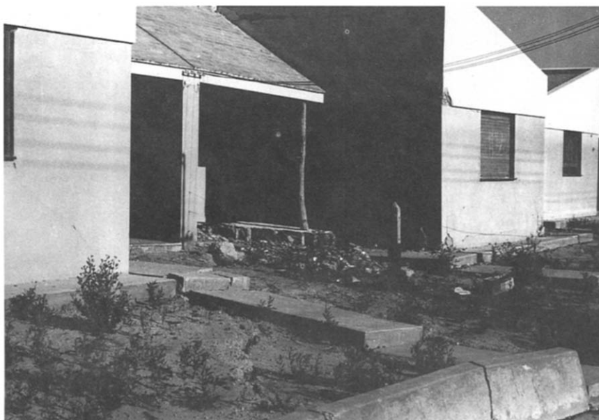
Fig. 5. House in Barrio J.C. Castro intersected by a ground fissure that pulled apart and vertically offset the slab foundation and cracked or collapsed exterior and interior walls. Note the cracked and tilted walks and curbs in the foreground and the collapsed wall of the house in the background.
