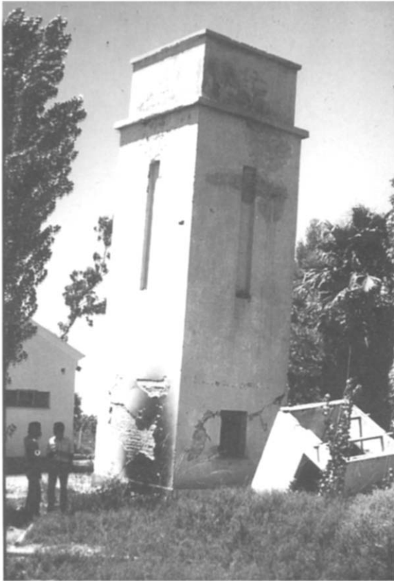
Fig. 17. Photograph of the water-storage tower that tilted due to loss of bearing strength and nearby pump house that toppled into an eroded crater.
