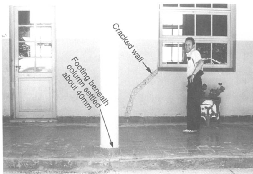
Fig. 23. Building at Escuela J.J. Pasos with cracked wall and differentially settled columns due to ground settlement and loss of bearing strength caused by liquefaction of subsurface sediments.
