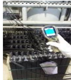
Figure 45 SUNLIGHT manual temperature monitoring procedure
