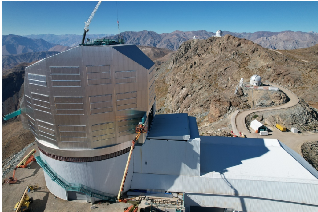
Figure 1.10: The Vera C. Rubin Observatory (foreground), as of April 2023. The Rubin Auxiliary Telescope (used for commissioning and measurements of atmospheric transmission) is up the road to the right of the Rubin dome. On the background ridge are the SOAR (left) and Gemini South (right) telescopes. Image credit: Rubin Observatory.
